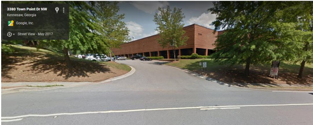
Entrance to S&MEs office
