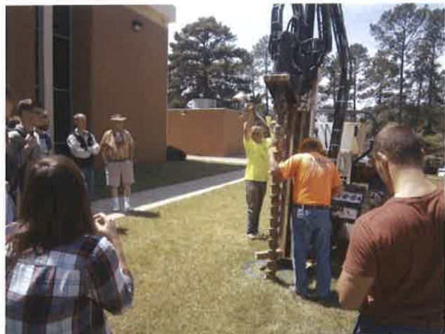
Hollow stem auger drilling
